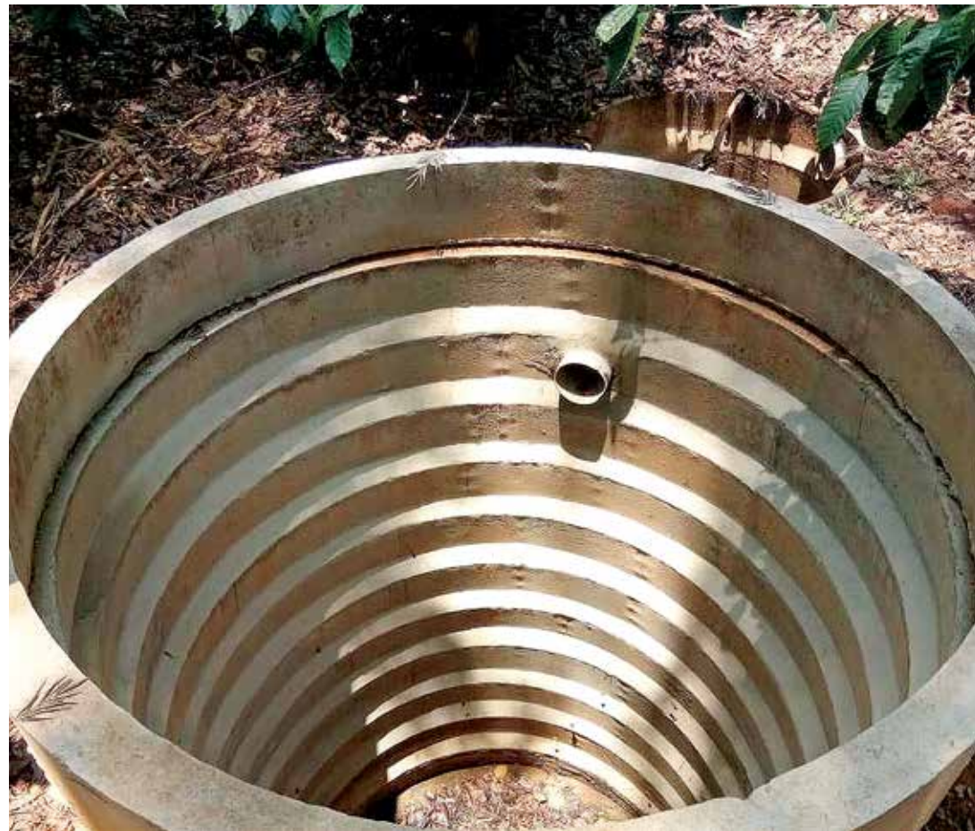
A typical recharge well
