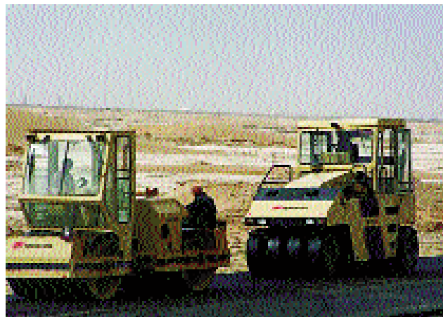
Road building in progress
