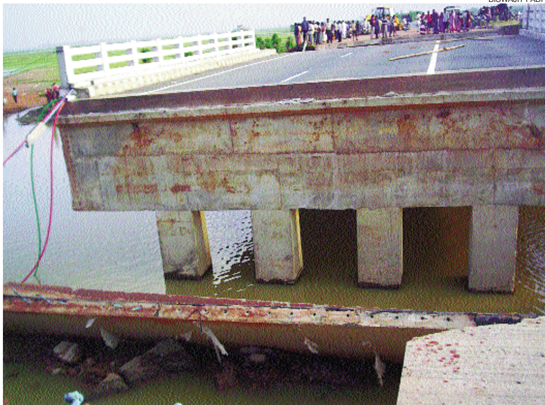
A bridge that caved in
