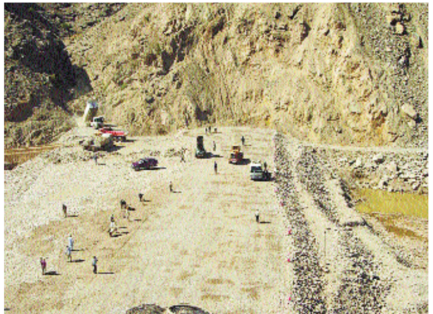
Construction of the Salma Dam
