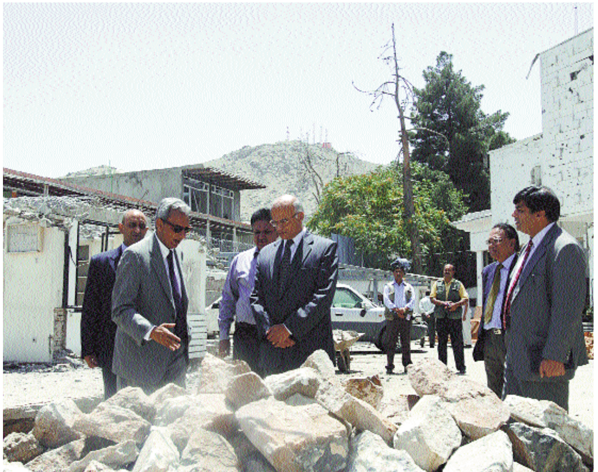
The Foreign Secretary at the damaged embassy in Kabul
