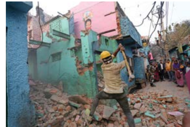
A worker from DDA knocking down a home
