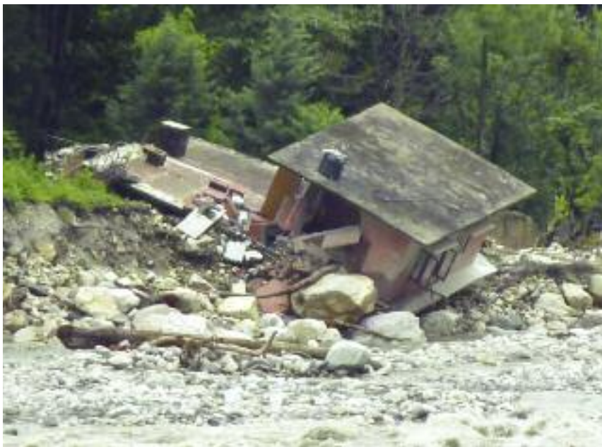
A house inundated by the recent floods in Uttarkashi
