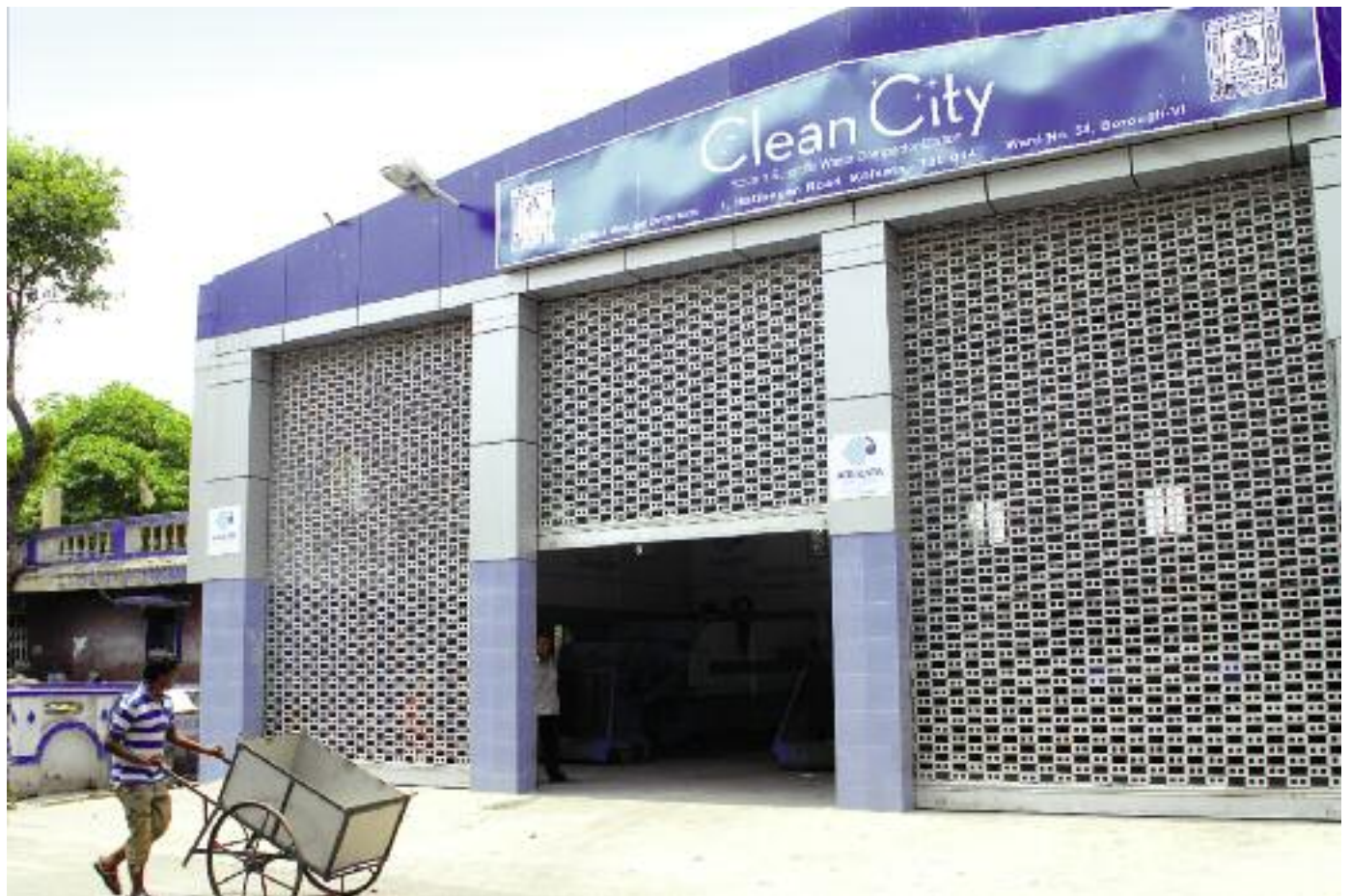
The problem with compactors is that they disallow segregation of recyclables
