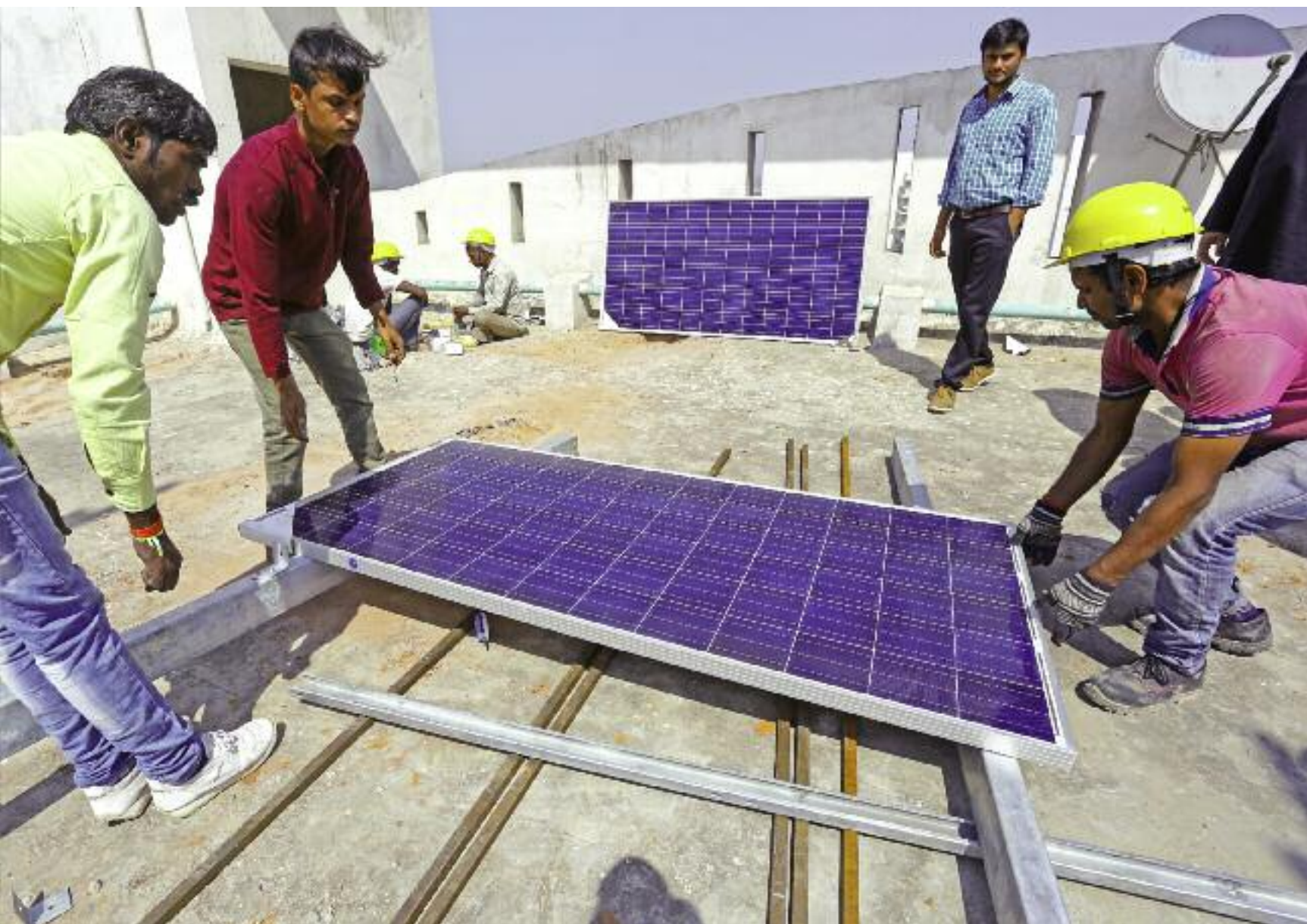
Solar panels being fitted on one of the rooftops at Bestech Park View Residency
