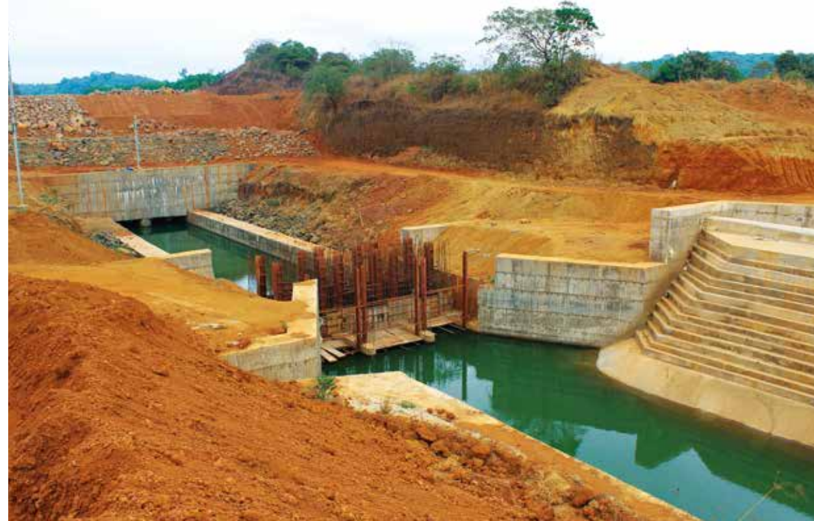
The aquaduct that has been built on the Kalasa river
