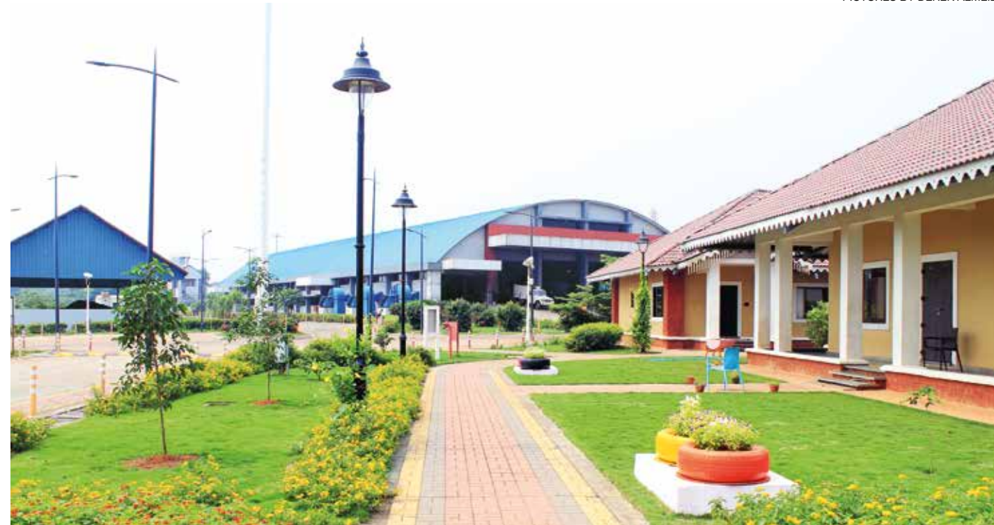
A view of the ₹140 crore waste treatment plant at Saligao
