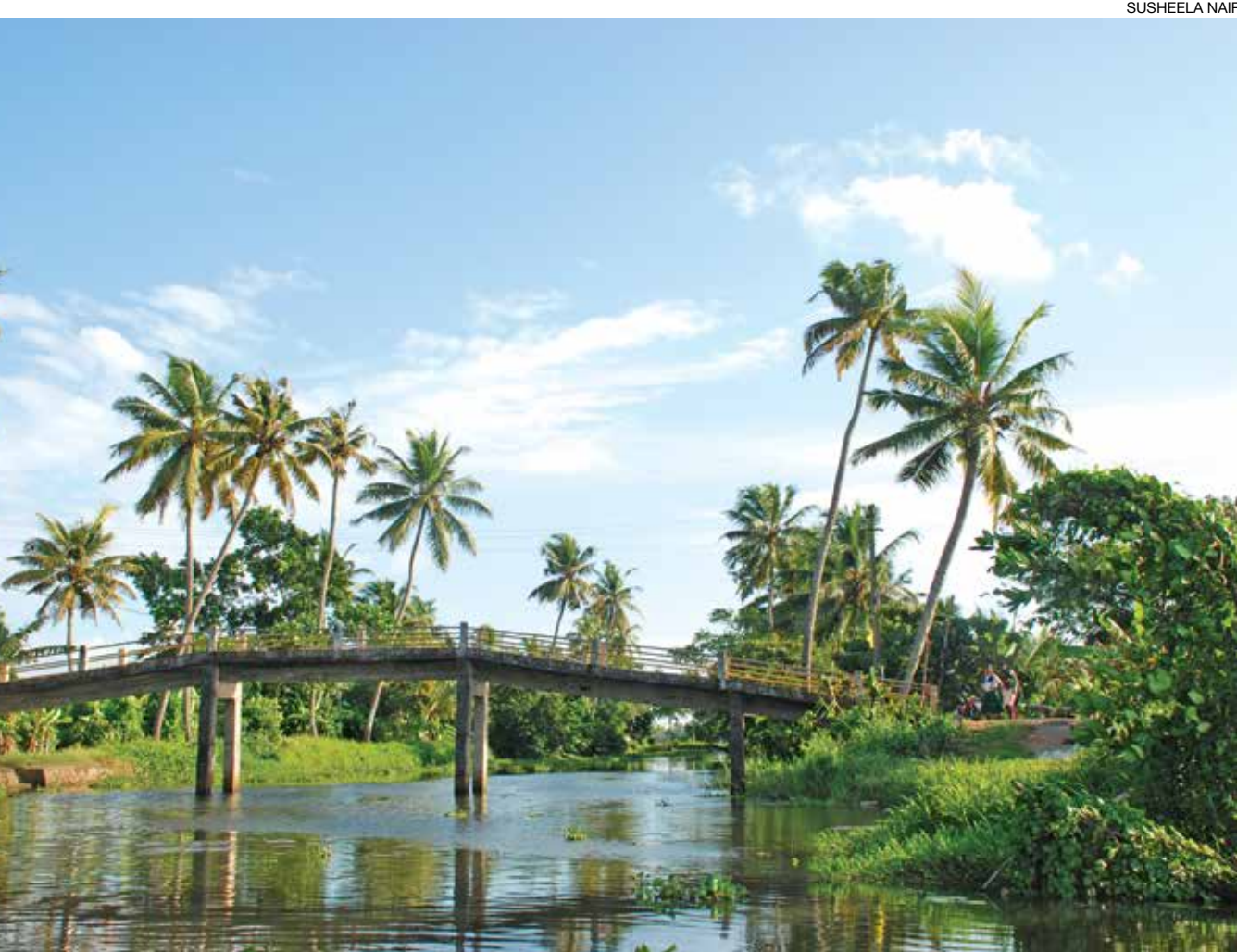
A bridge across the backwaters of Kumarakom
