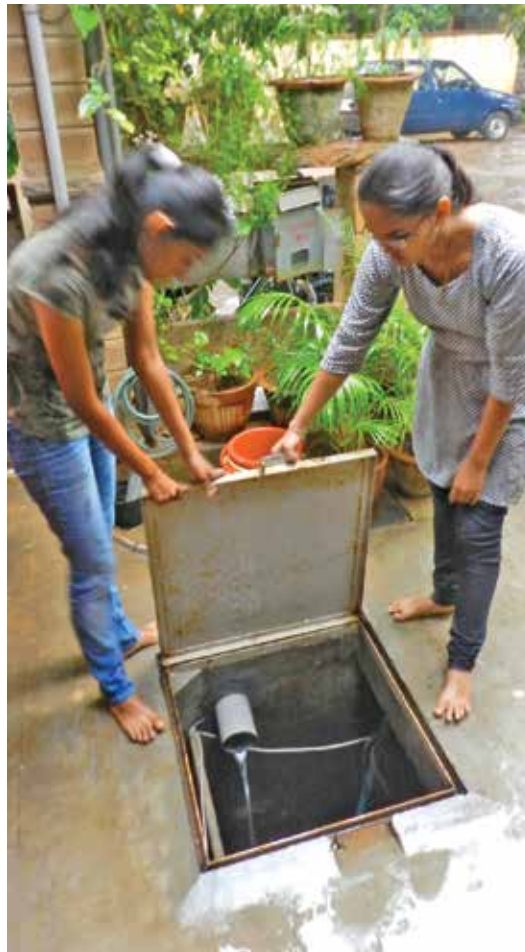
Harvesting rainwater isn't difficult or costly
