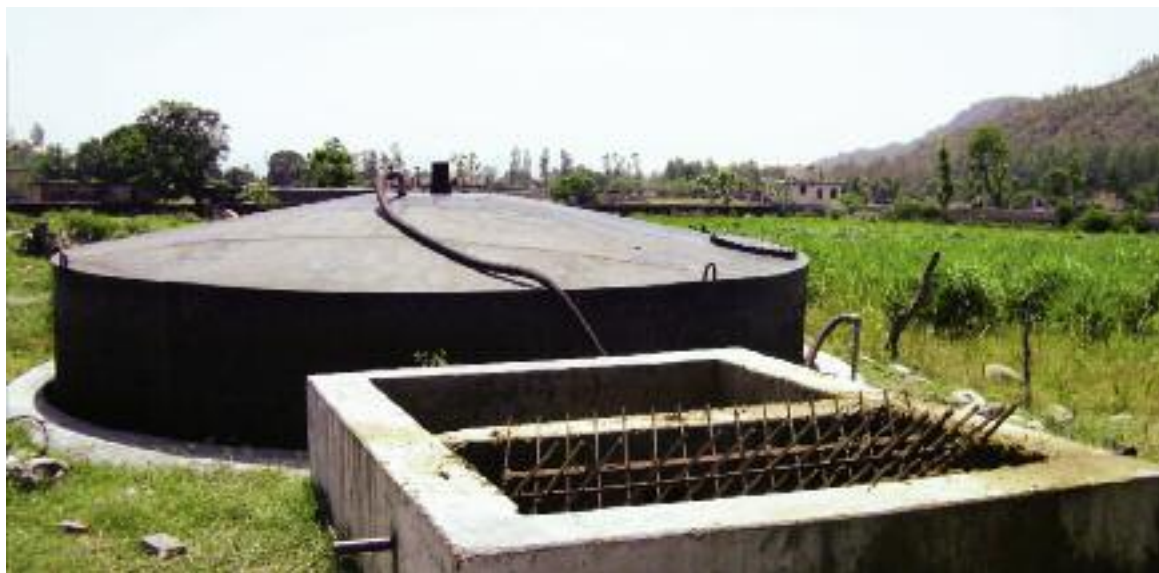
AFBC's biogas plant produces electricity from cowdung
