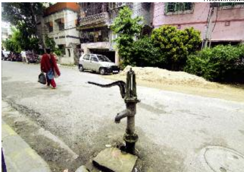
A tubewell with arsenic in its water at Lake Gardens in Kolkata
