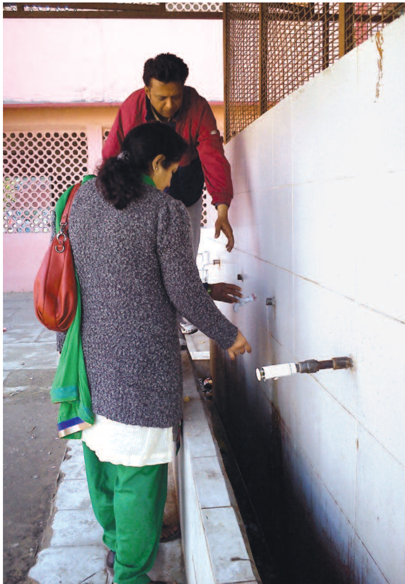
AAP volunteers examining new taps that have been installed in schools
