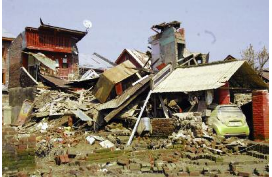
Houses have been reduced to rubble
