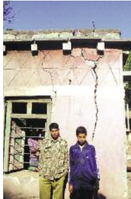
Homes have cracked walls and leaky roofs
