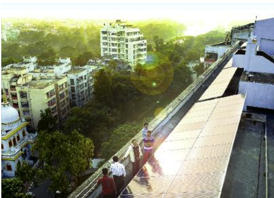
View of the SIRSA apartment block's roof
