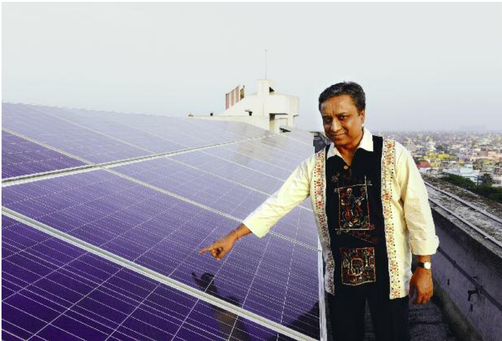
Avijit Ghosh with the rooftop solar panels installed at the SIRSA apartment complex and guest house
