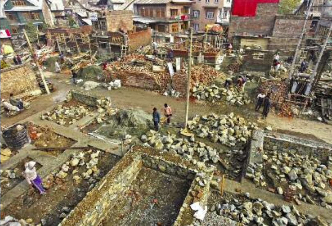
Residents have not been able to rebuild their homes damaged by the floods
